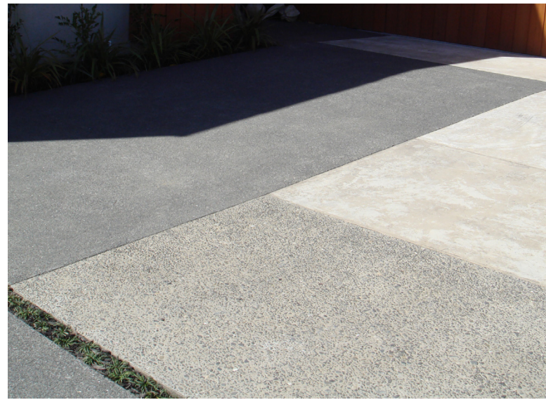
1. Mixed in-situ concrete circulation paths with coloured oxide finish to prevent glare and stamped edge
