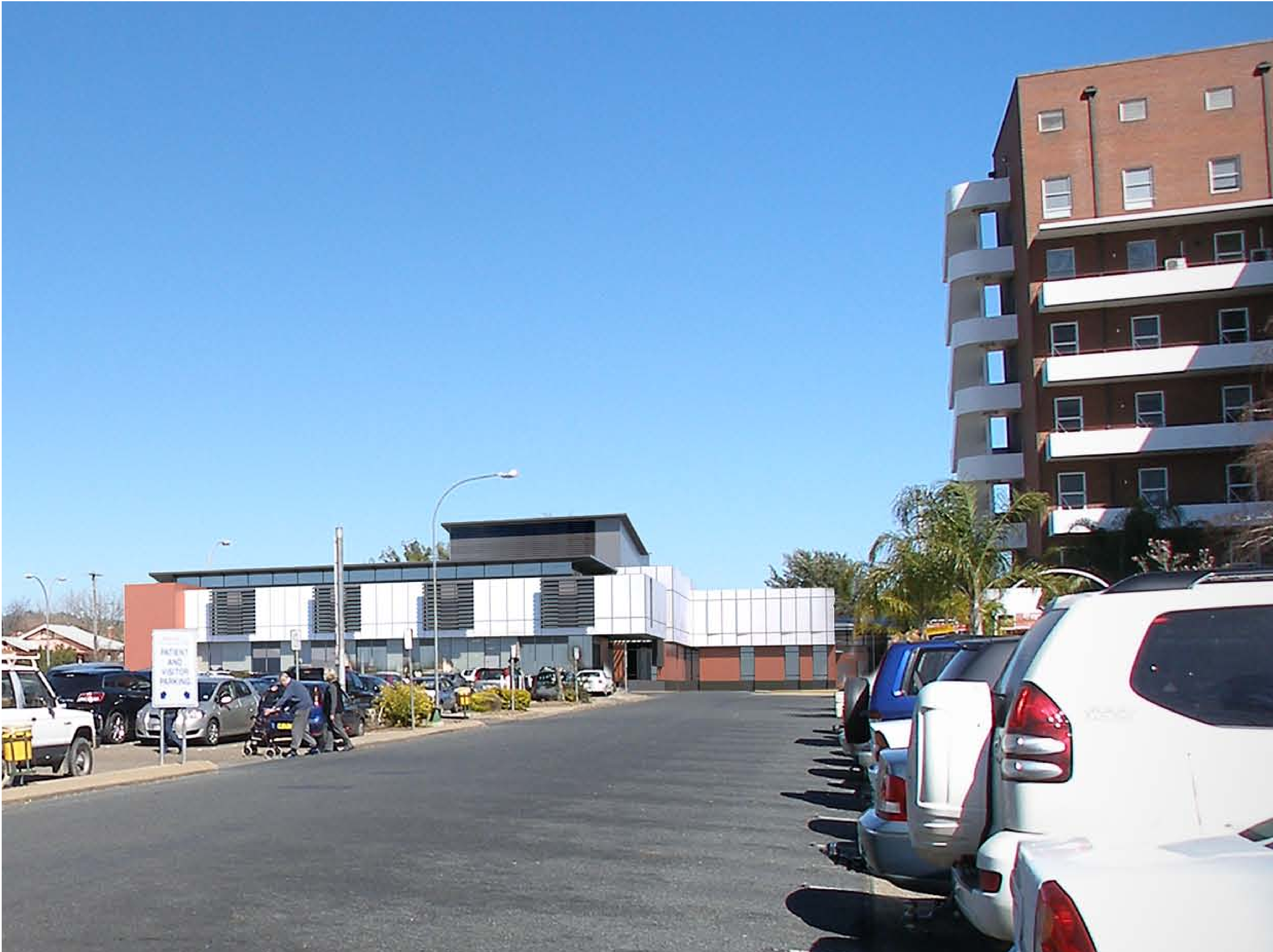
1 NORTH VIEW DOWN LEWIS DRIVE NTS
