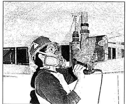
Concrete drill with a HEPA filter attachment.
