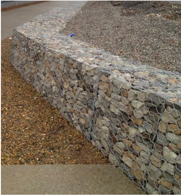
BRICK PIT PARK - GABION WALL & EXPOSED AGGREGATE PATH
