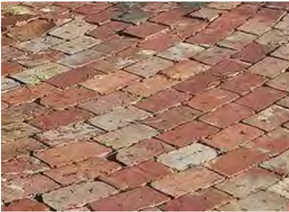
RECYCLED RED BRICK PAVING. CRUSHED BRICK IN TREE PITS.
