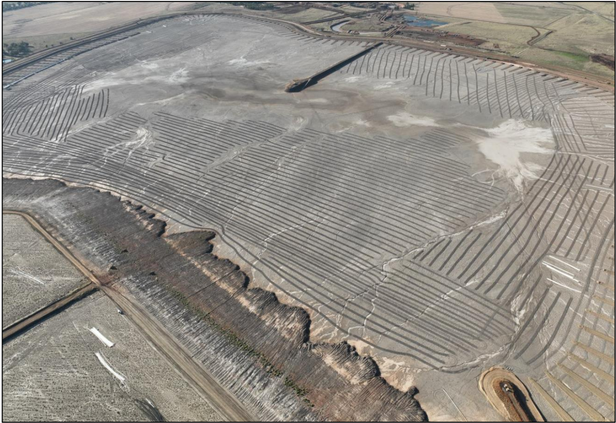
Figure 9 Ripping undertaken on Rosedale TSF for dust control
