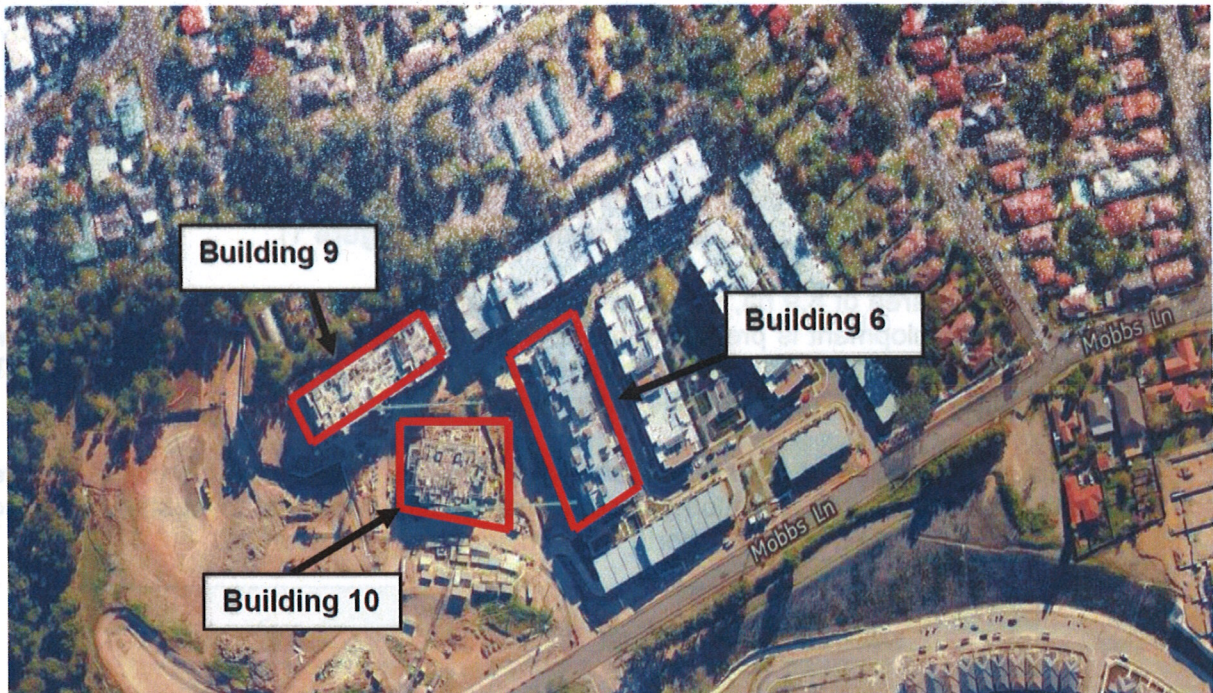
Figure 2: Aerial View Identifying Buildings 6, 9 and 10
