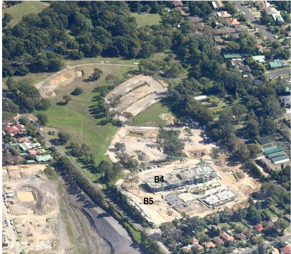
Figure 6: Subject site, currently under construction. Buildings 4 and 5 in the foreground
