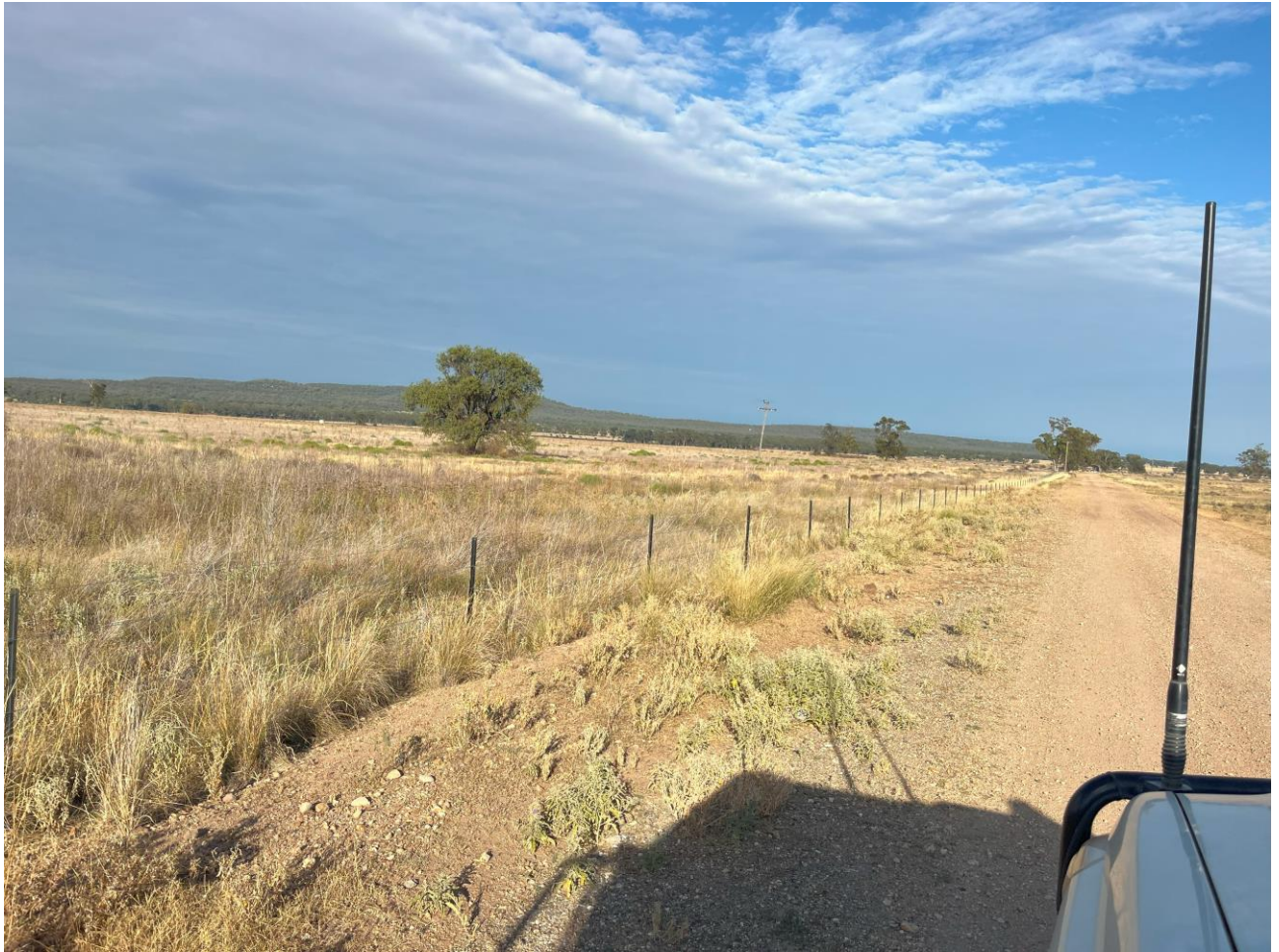
New Fencing typical of various locations.
