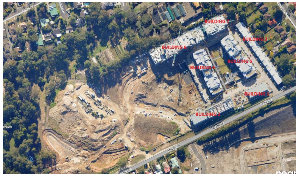
Figure 6: Subject site, currently under construction
