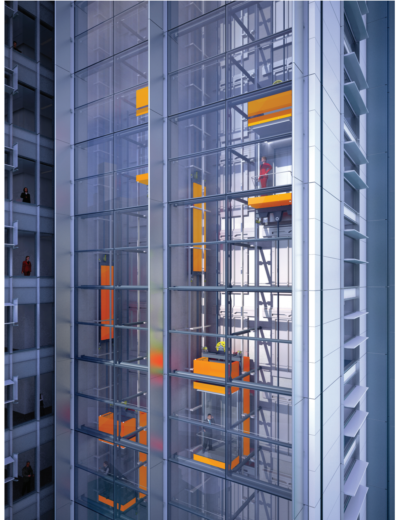
Glazed Lift Shaft: View of the glazed lift shaft, the neutral colour strategy of the steelwork and facade elements contrasts with the dynamic and boldly coloured lift cars and counterweights.
