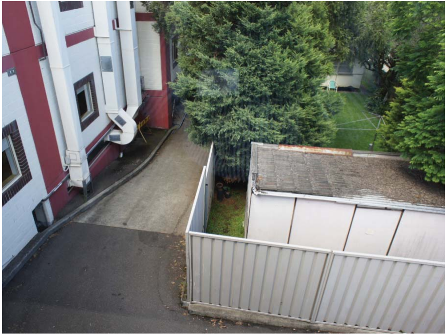
VIEW 4: EXISTING PHOTO
