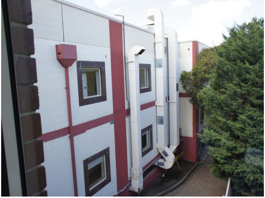
VIEW 3: EXISTING PHOTO
