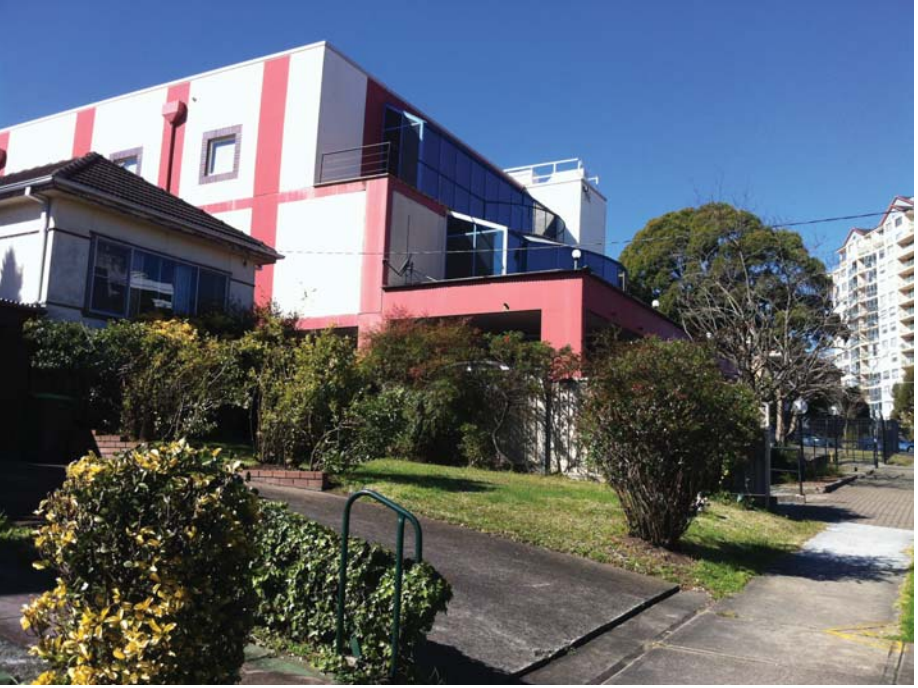
VIEW 2: EXISTING PHOTO
