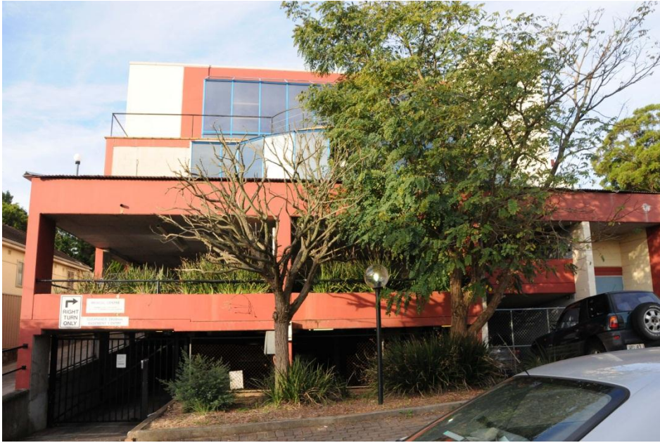
FIGURE 7: BASEMENT CAR PARK FROM MILLETT STREET
