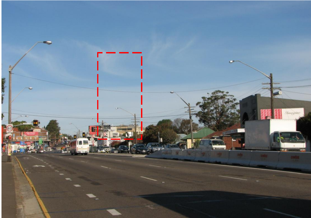
Motorist Position: Victoria Road after cnr Terry Street
