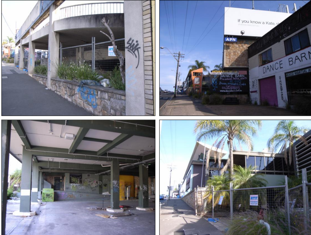
Figure 8: Above the Victoria Road buildings comprising the Dance Barn and Balmain Leagues Car Park and Club building.
