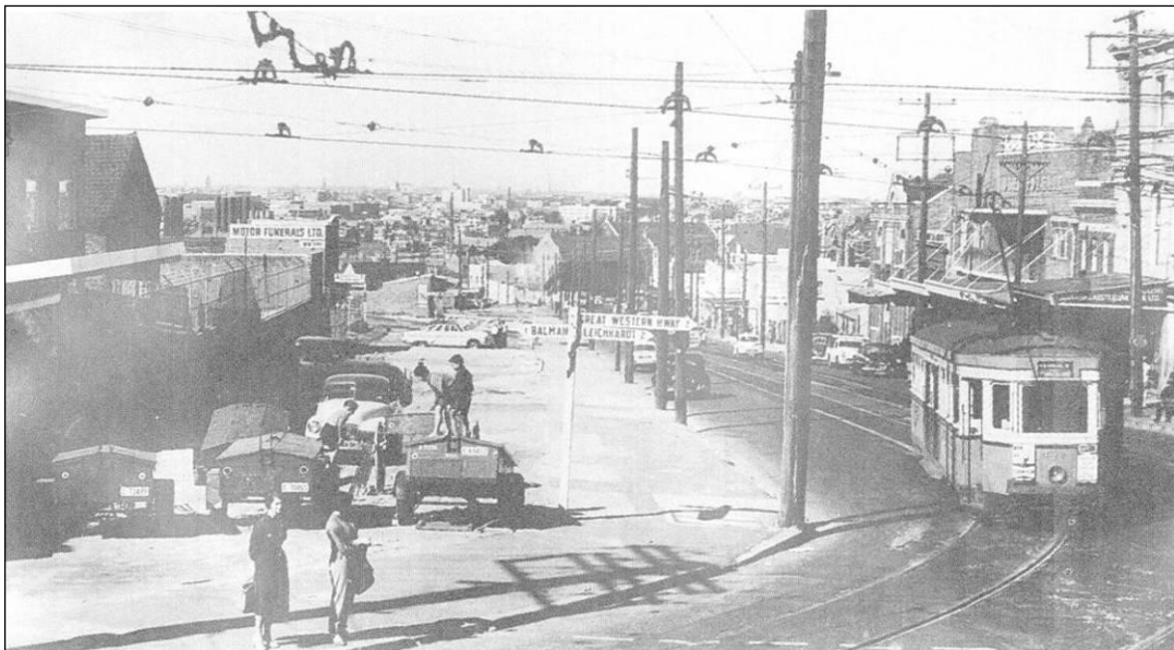
Figure 21: View from the corner of Darling Street and Victoria Road, looking south east and showing the impact of the widening of what was Weston Road for Victoria Road. The photograph is dated late 1950's- early 1960's. This view is diagonally opposite the subject site.
