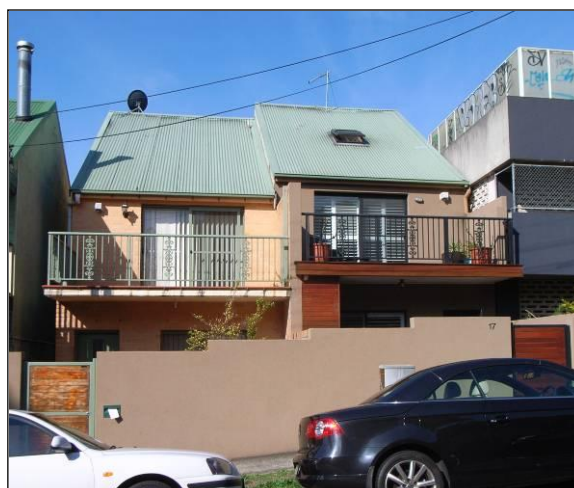
Figure 6: The recently constructed pair of stepped terraces at 17 - 19 Waterloo Street Rozelle, located next to the two level carpark shown above.
