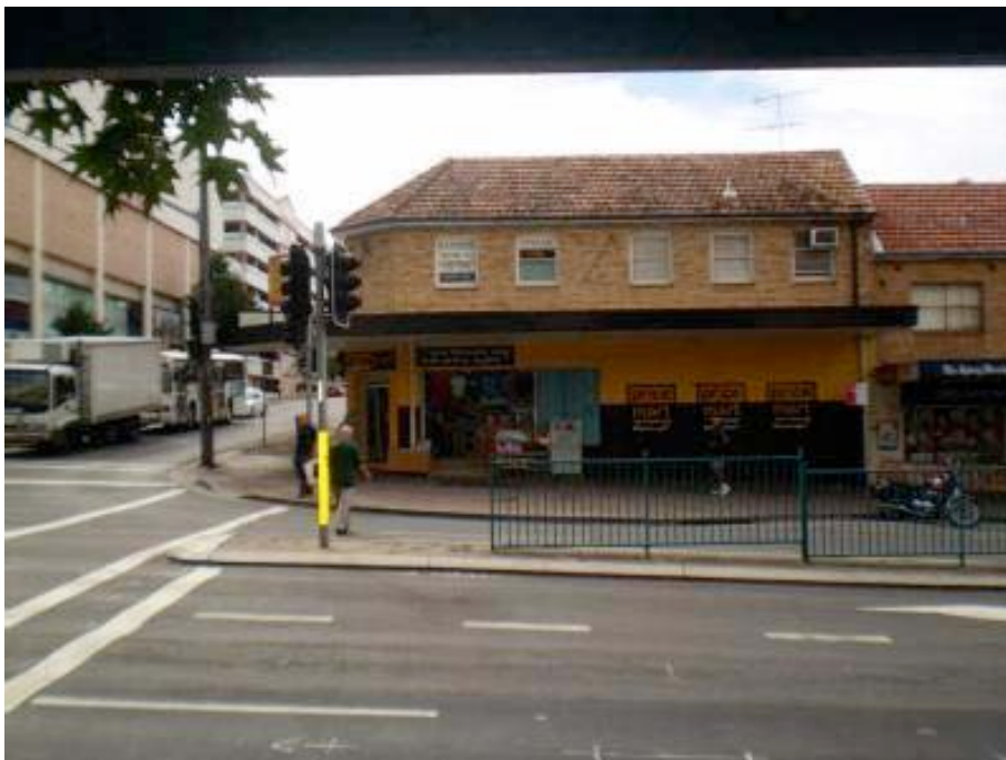
Figure 7 – View of the Existing Building from the West
