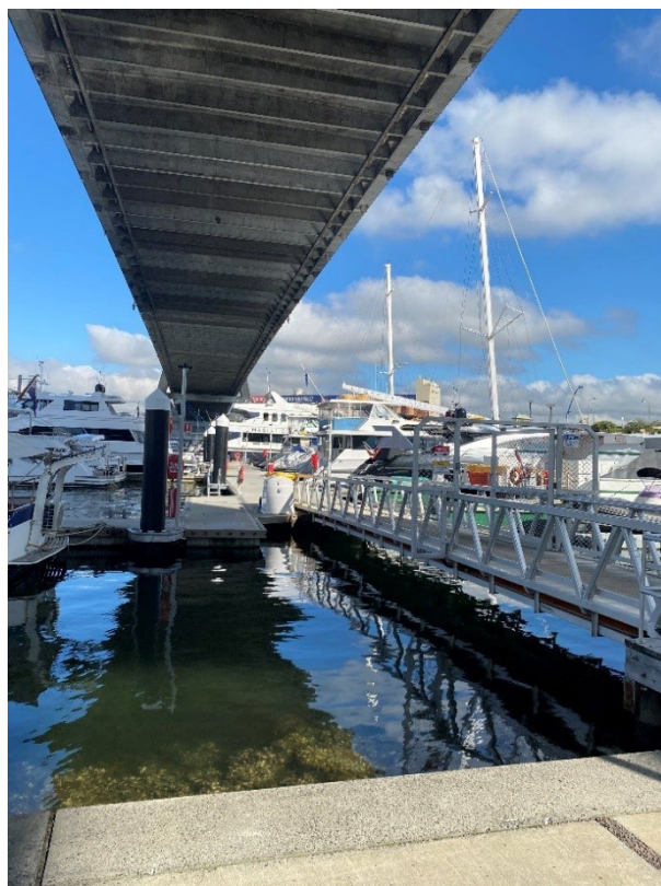
Figure 3 | Existing moorings under the ANZAC Bridge looking west
