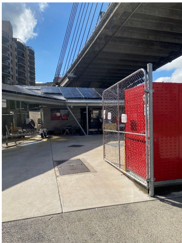
Figure 2 | Existing temporary building for the Blackwattle Bay Marina looking north-east
