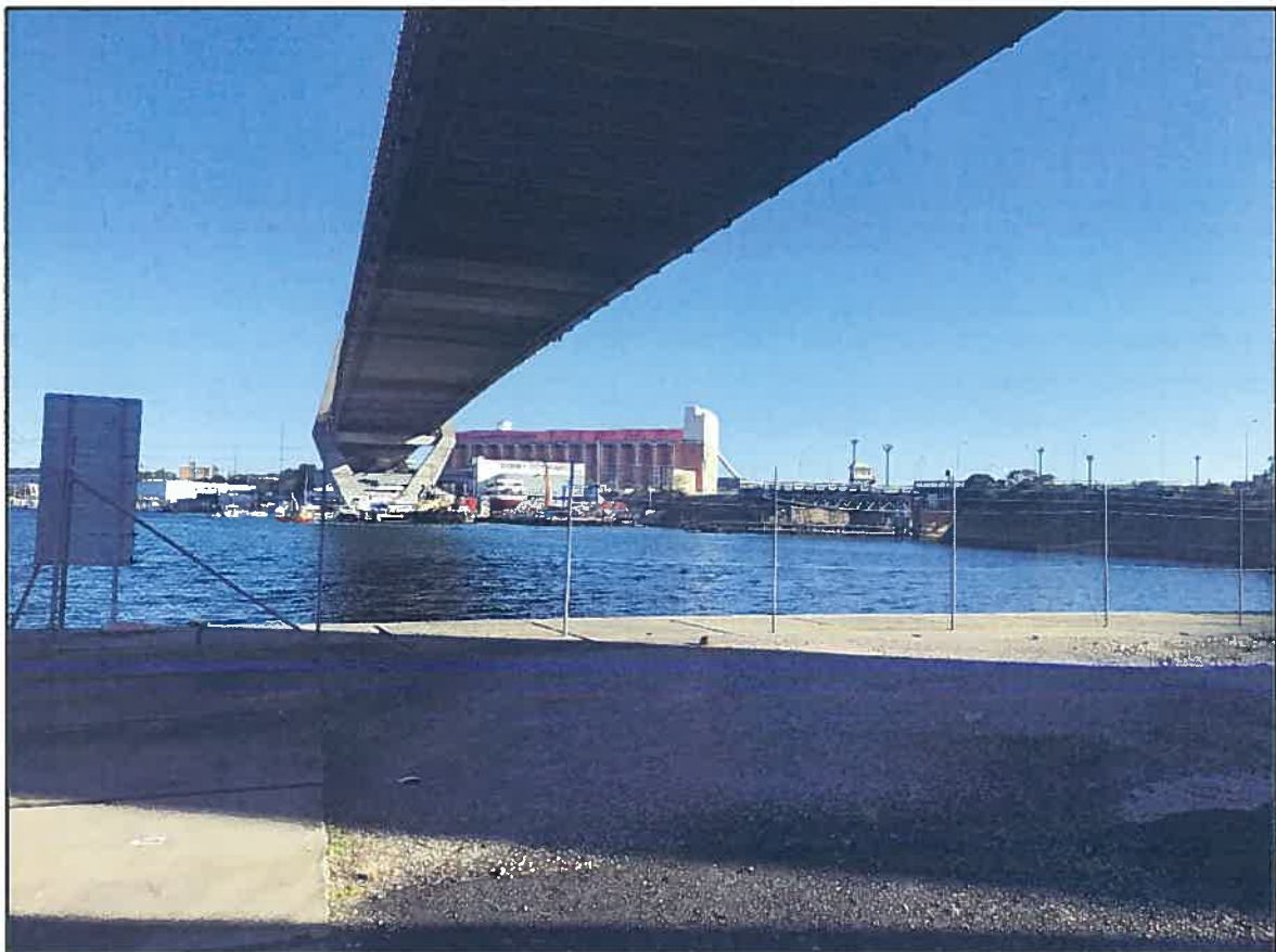
Figure 2 | Looking west from the site to the Glebe Island Bridge and working harbour uses of Rozelle Bay (Base source: DPE photograph)
