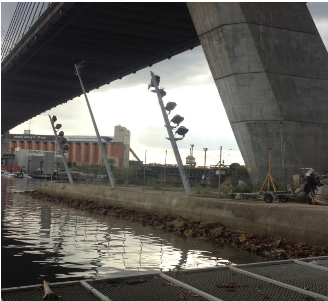
Figure 9 – Seawall at the site viewed from passive (dragon boat) ramp
