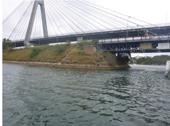
Picture 21 – The southern bridge approach (adjoining the subject site)
