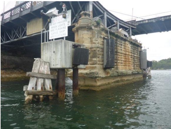
Picture 22 – Detail of the bridge pylon
