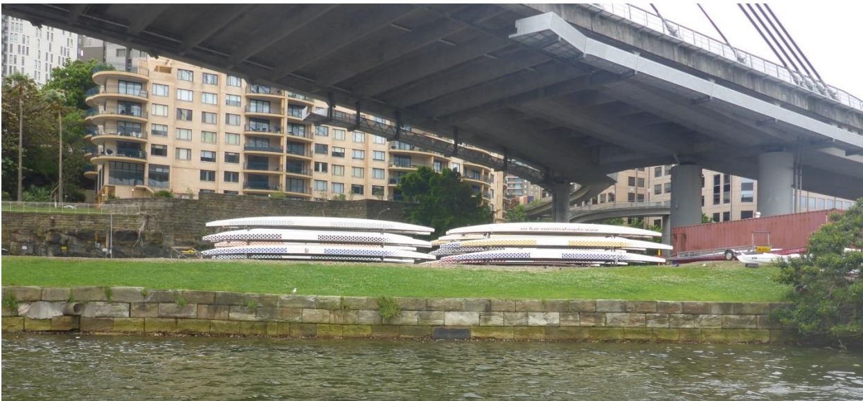
Figure 2 – Views of the subject site from Blackwattle Bay
