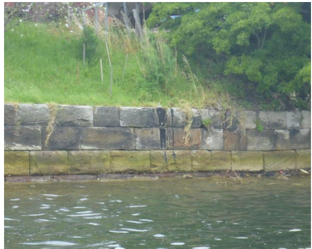
Picture 8 - Detail of the seawall
