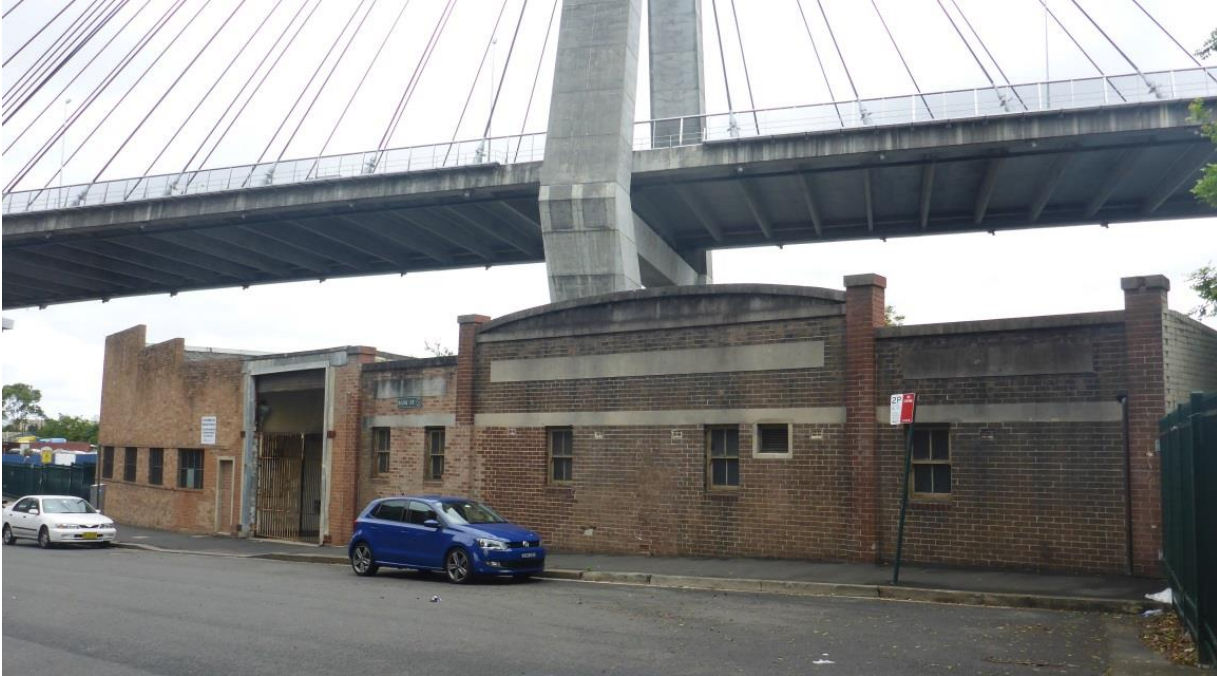
Picture 9 - The northern building is the earliest extant building on the site, with the fabric suggesting an early inter-war construction
