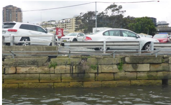
Picture 16 - Fish market carpark and sea wall
