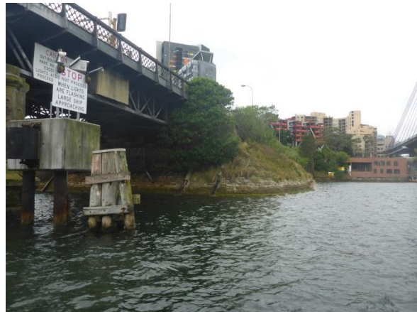
Picture 23 – View towards the subject site from the bridge/ Blackwattle Bay
