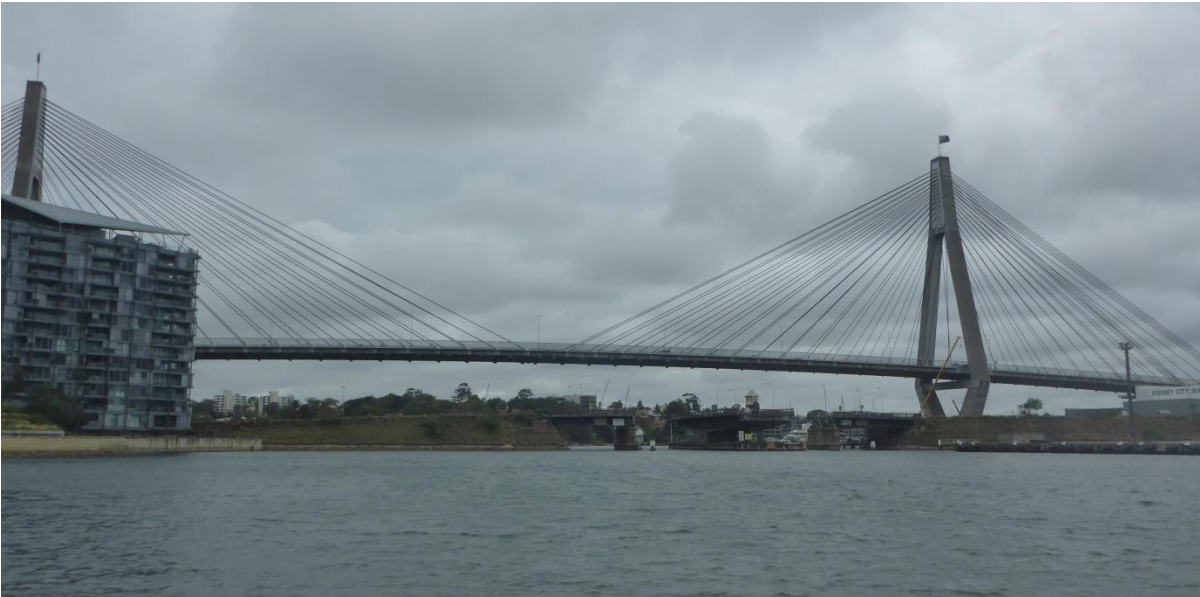
Picture 24 - View of the bridges spanning Johnstons Bay
