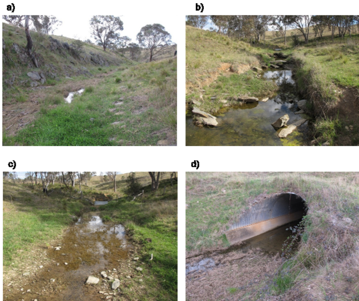
Plate 4: WPT 339: a) Downstream view; b) Upstream view; c) Further upstream; d) Existing culvert.
