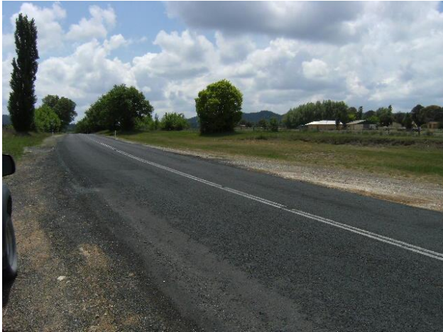
Looking north east across area of known surface NOA
