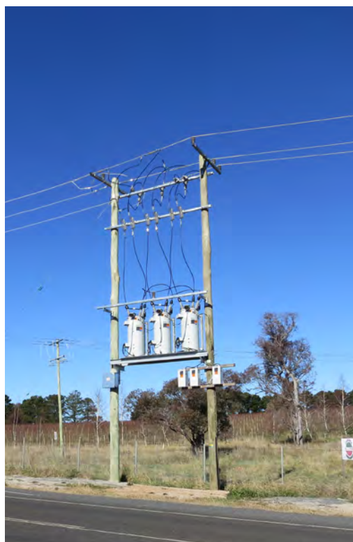
Photo 02 - Proposed voltage regulator
