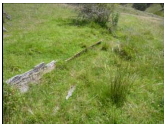
Figure 7.35 Section of water race with u-shaped timber.
