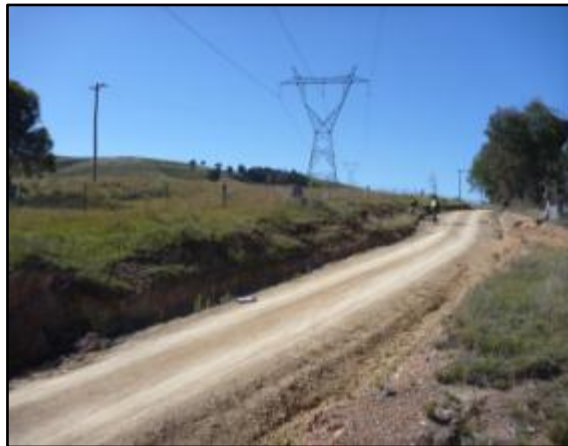
Figure 7.1 Oaky Creek 1 looking southeast
