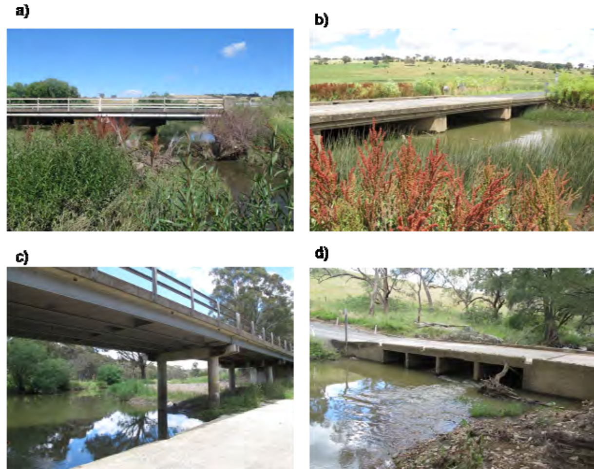
Plate 4: Summer Hill Creek Crossings: (a) First Crossing; (b) Second Crossing; (c) Third Crossing 3; (d) Fourth Crossing.
