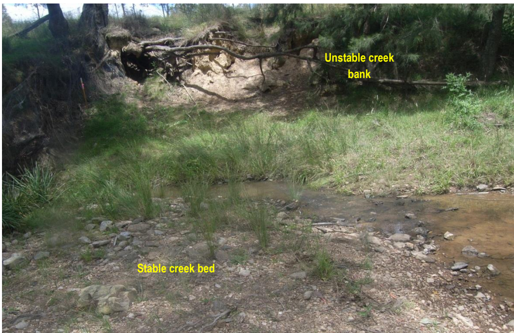
Figure 5-4: Oaky Creek – active erosion on right bank downstream of causeway
