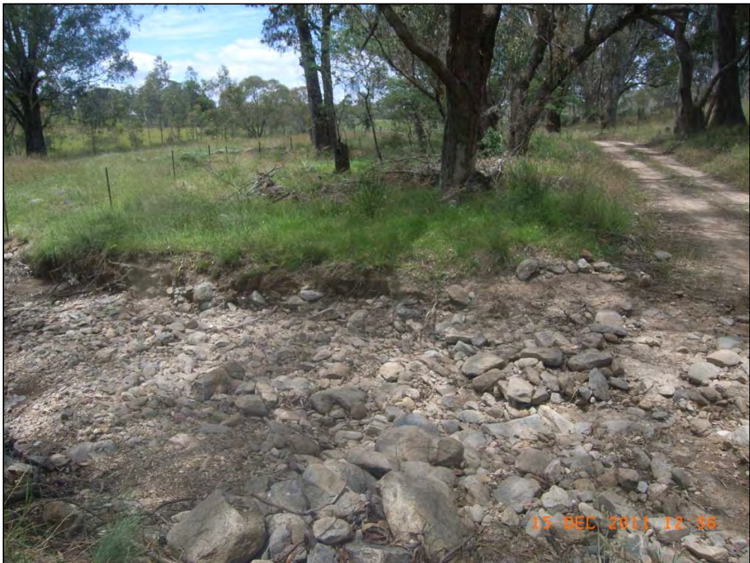
Figure 20 Looking to the right bank from the left. Note the road surface is integrated into the creek bed. Note the slight grading up to top of banks and exposed soil on upper bank.
