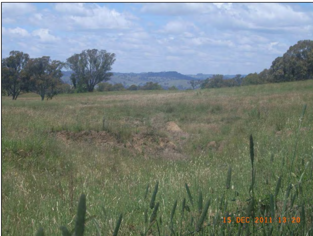
Figure 15: Looking upstream from Lookout Road. Gully formations at least 100m upstream of the road culverts obvious sign of previous bank erosion. The creek channel appears to have restabilised.
