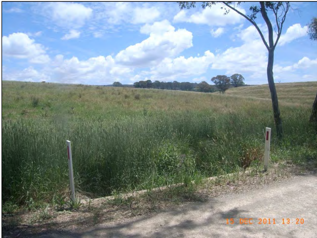
Figure 14: Looking downstream from Lookout Road. Well grassed shallow channel with a silt and clay bed material.
