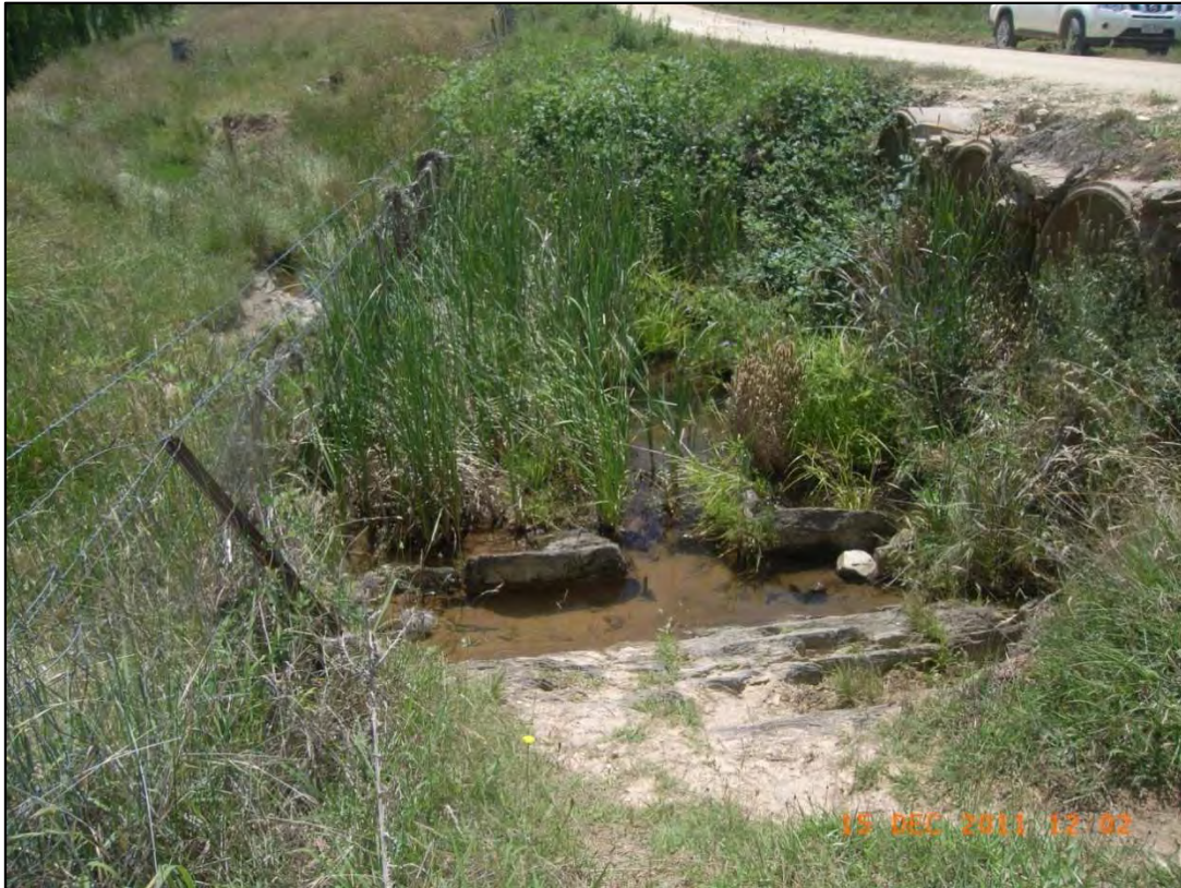
Figure 21 Downstream side of Long Point Road looking from left bank to right. Note the channel material of bedrock, boulders, silt & clay with in-stream vegetation and grasses/shrubs on the banks.
