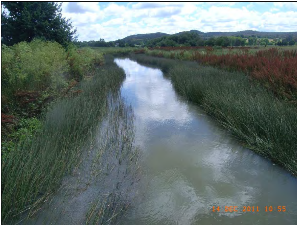
Figure 3: Looking downstream at Crossing 2. The banks are well vegetated, though the channel width is a lot smaller than for Crossing 1, resulting in higher velocity flow. Sit and Clay bed material with little deep rooted vegetation/trees.
