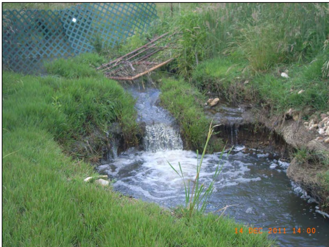
Figure 13: Looking upstream from Ophir Road at head-cut and plunge pool, most likely a result of the road crossing construction changing the bed level and hydrology of the creek.
