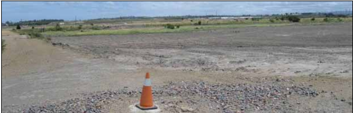
Photo 27: Site D - looking south-west from the northern boundary of Cell 2 in the FDF (January 2011)
