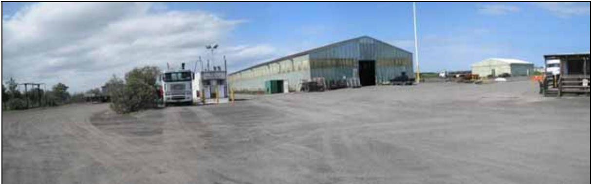
Figure 6: Diesel bowlers and aboveground tank in western portion of Site F, looking north to north-east (December 2011)
