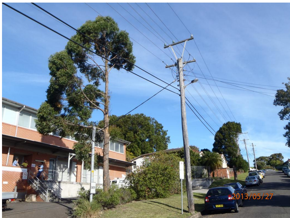
Plate 4: Image showing Tree 6 and the extensive pruning for wire clearance. P. Vezgoff.
