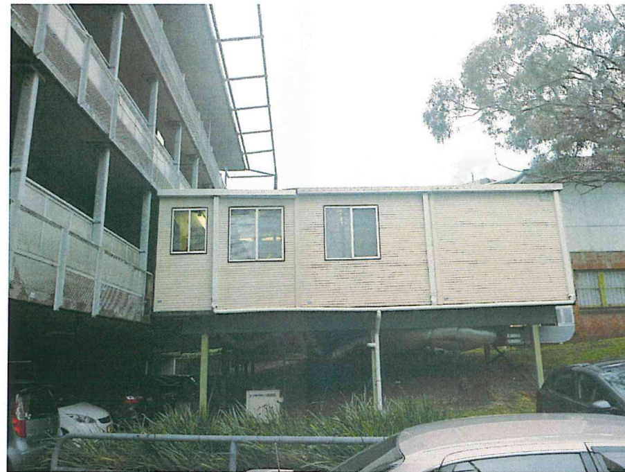
PHOTO 2 - WEST VIEW OF EXISTING DEMOUNTABLE BUILDING FROM ON-GRADE CARPARK
