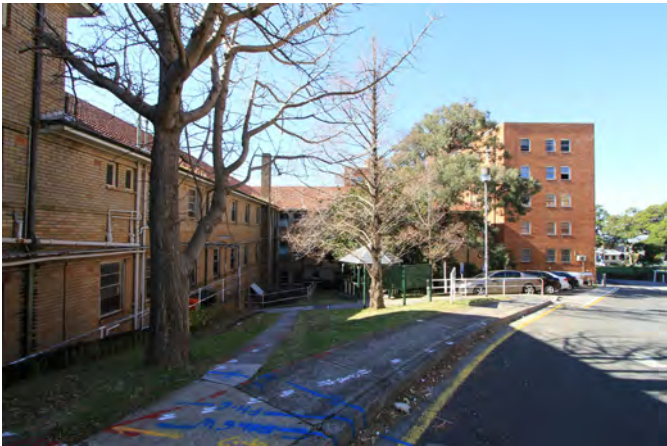
Rear of Elouera House and Hospital Road
