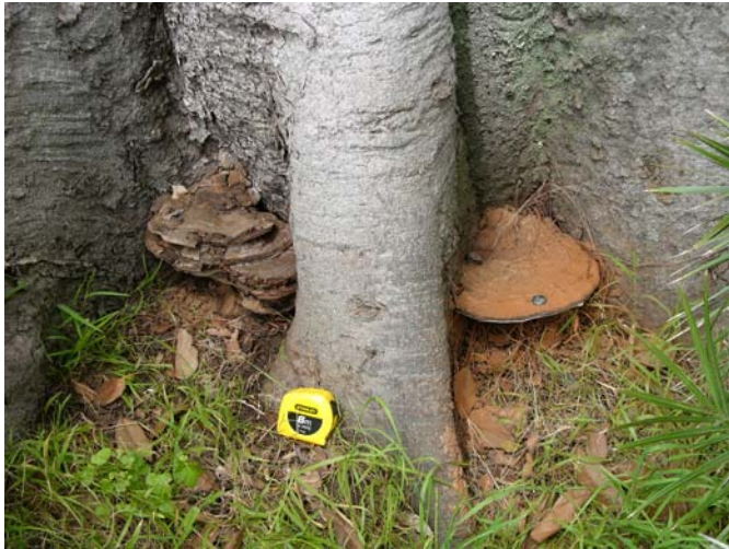
Plate 1 - T1 (Moreton Bay Fig) showing large fruiting bodies of Ganoderma sp (Ganoderma Butt Rot) on lower trunk.
