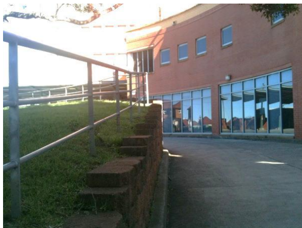
Figure 5.11 Retaining wall adjacent to Hospital Road, showing extent of excavation here. (Source: GML 2011)
