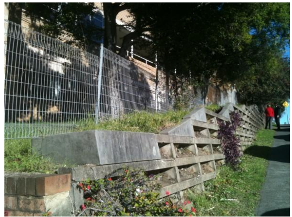
Figure 5.4 Retaining wall along Loftus Street adjacent to Elouera House showing extent of excavation. (Source: GML 2011)
