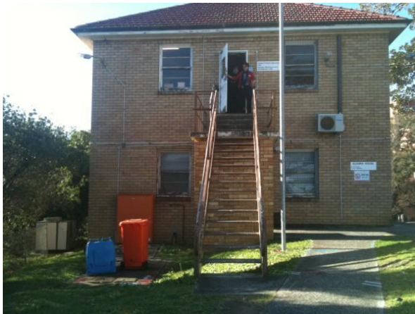
Figure 5.1 Elouera House, view east, showing differences in ground levels. (Source: GML 2011)
