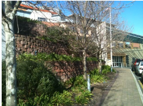
Figure 5.8 Retaining wall at Loftus Street entrance showing extent of excavation and filling. (Source: GML 2011)
