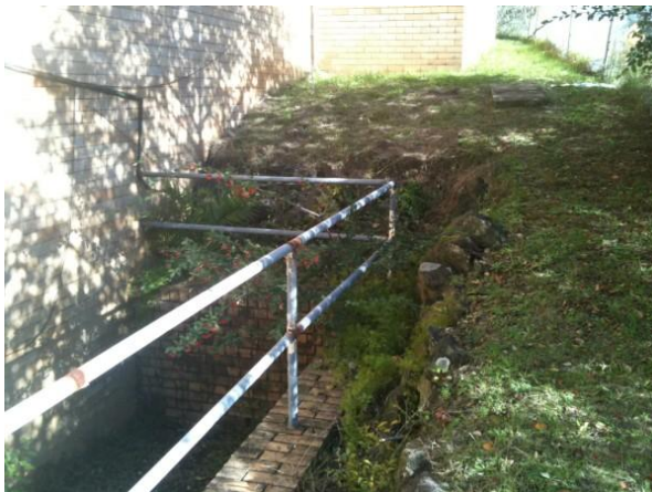
Figure 5.3 Retaining wall adjacent to Elouera House. Note extent of excavation present. (Source: GML 2011)
