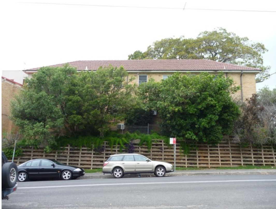
Figure 2.2 Street elevation of 1941 wing of Elouera House, by Government Architect Cobden Parkes (Source: GML 2010)
