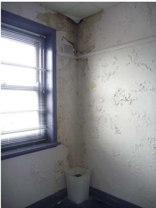
Figure 3.24 Water damage and signs of a leaking roof in the former study and library (now TV room). (Source: GML 2011)
