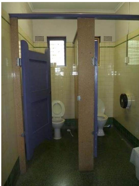
Figure 3.28 Original toilet fit-out, with glazed ceramic tiles and terrazzo flooring. (Source: GML 2011)
