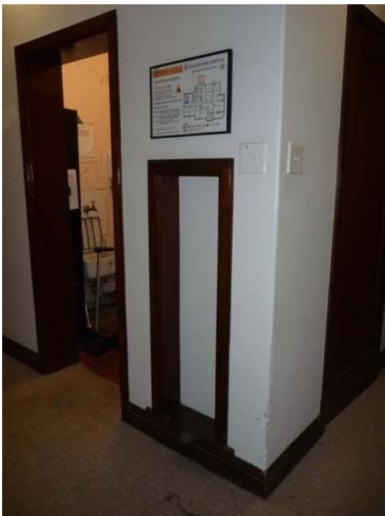
Figure 3.18 Purpose-built stand for a fire hydrant, constructed to match the skirtings and door frames. (Source: GML 2011)
