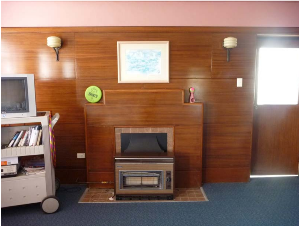
Figure 3.20 The sister's sitting room, showing intact original features including the fireplace and surround, tiled hearth, light fittings and timber panelling. (Source: GML 2011)
