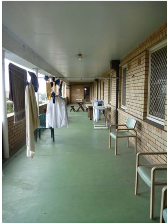
Figure 3.17 The first-floor balcony. The original drawings indicate that the balconies were to be laid in green silicate paving. The current finish is painted concrete. (Source: GML 2011)
