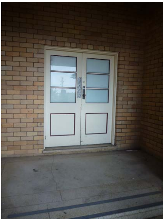
Figure 3.14 The front doors, constructed of painted timber. (Source: GML 2011)
