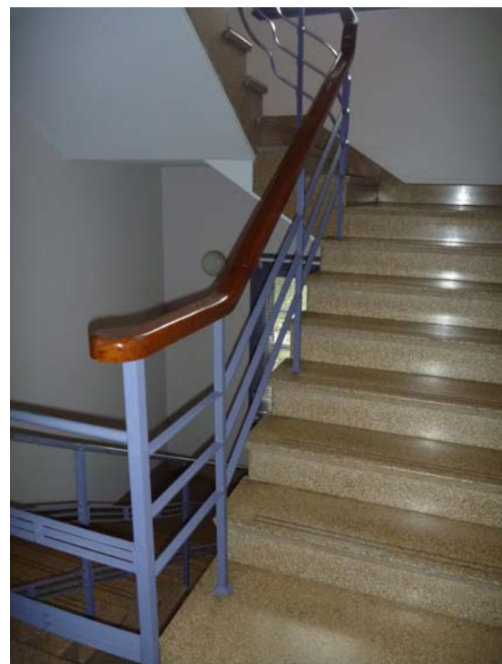
Figure 3.29 The later balustrade in the staircase to the 1941 extension. It is less elaborate than the earlier balustrade and has a timber top rail. (Source: GML 2011)
