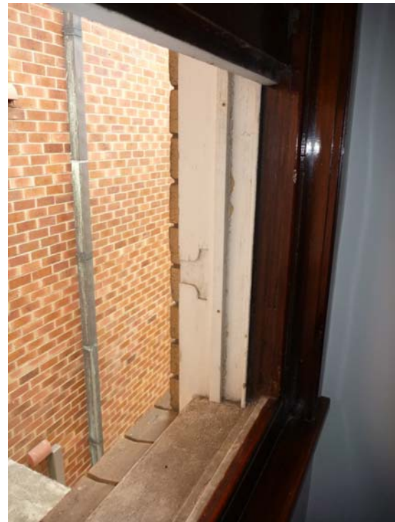
Figure 3.27 Evidence of the shutters that were once fitted to the windows along the east and west facades of the building. (Source: GML 2011)
