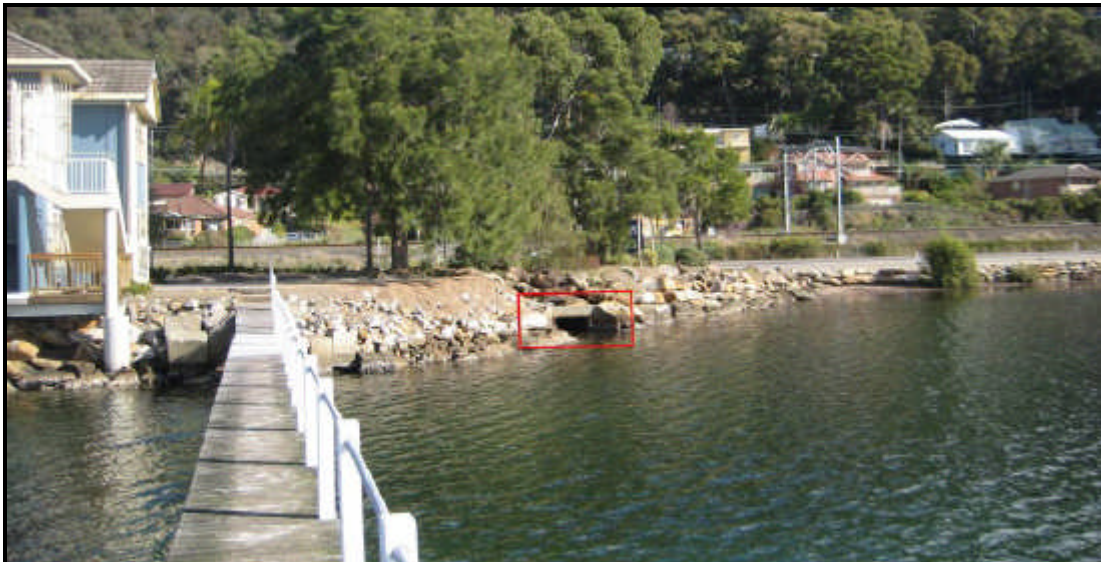
Figure 9: Looking back along the jetty to existing stormwater outlet
