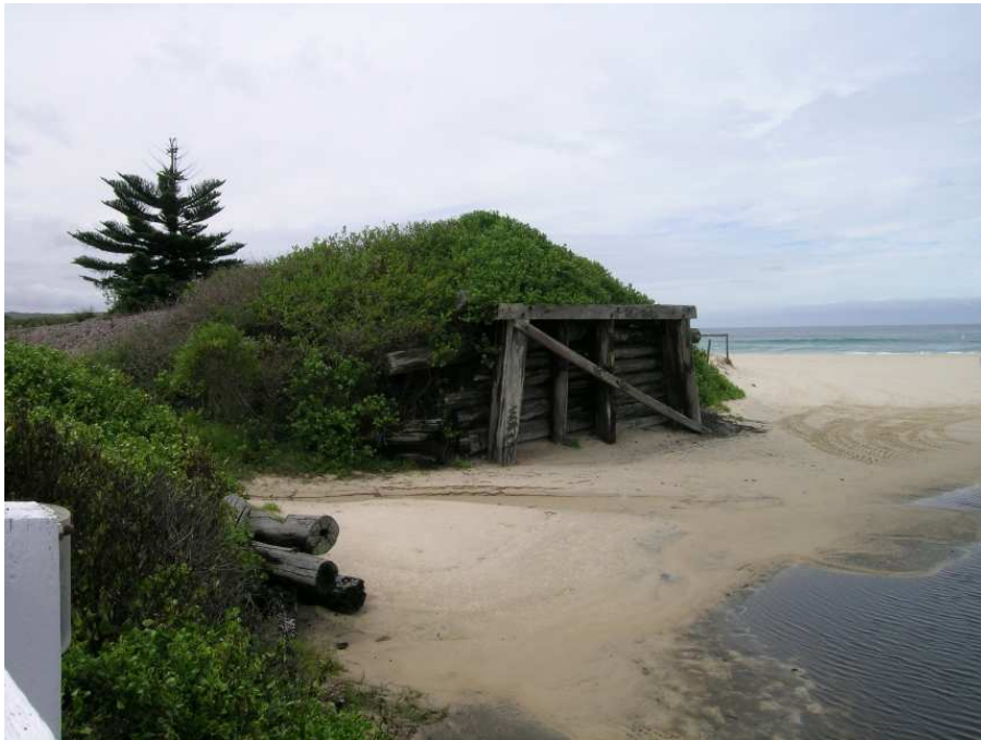
Fig.10 Remains of a bridge abutment, part of the former Colliery Railway
