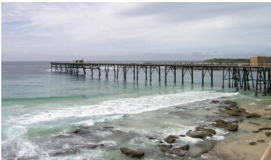
Fig.9 The Coal Loader Jetty
