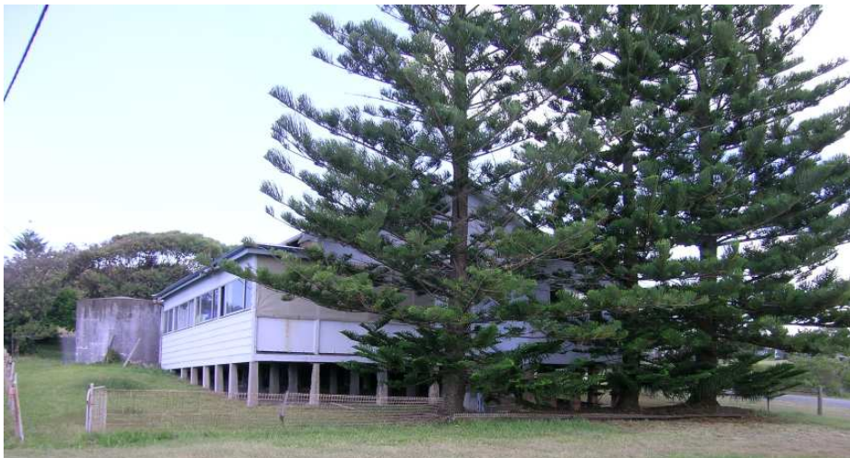
Fig.8 The Jetty Master's Cottage and stand of Norfolk Island Pines
