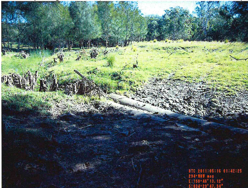
Figure 5 – Location of Reed Creek in the vicinity of the wastewater pipeline crossing showing previous disturbance (clearing for easement, culvert installation works and informal access point)
