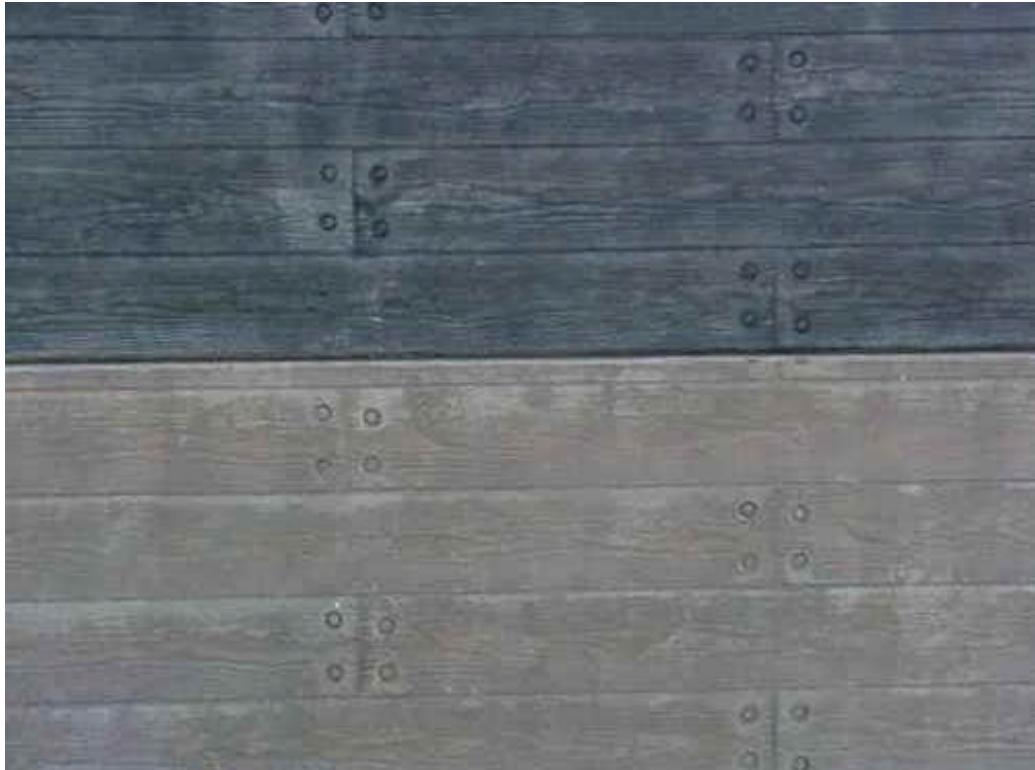
Demonstration Panel – Prestressed Concrete panel Cobblestone pattern
