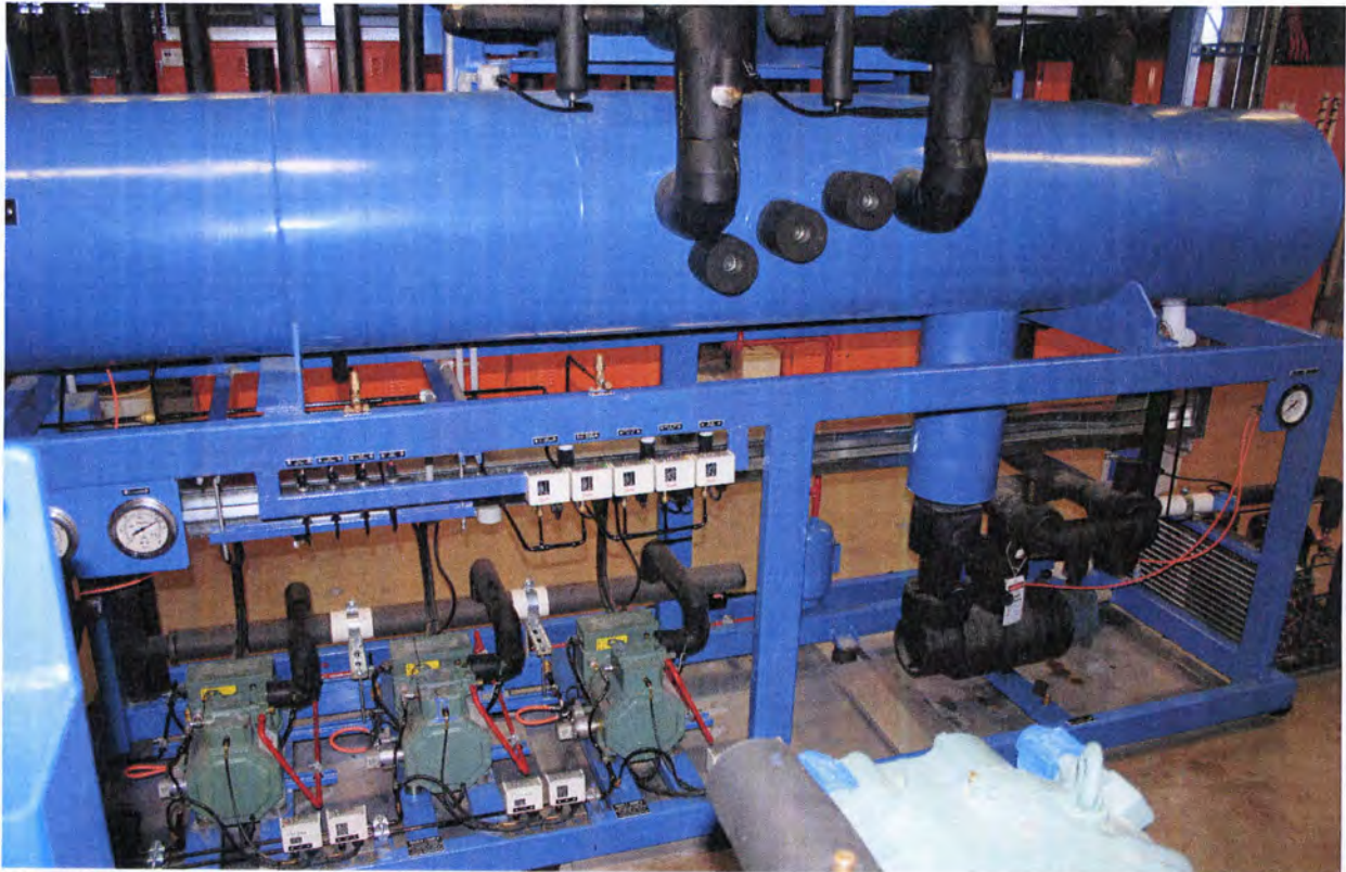
CO 2 Refrigeration Rack – Woolworths Norbrik
