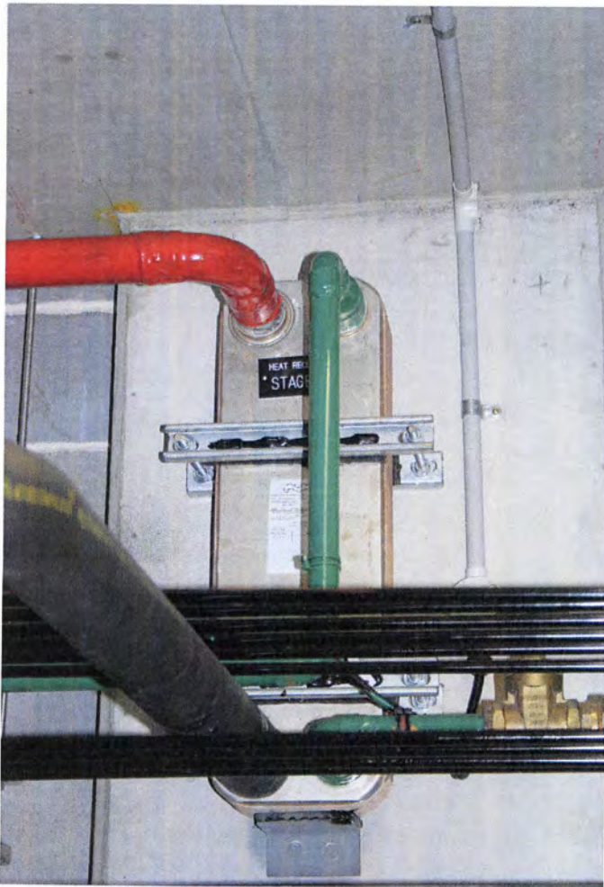
Heat Reclaim System – Woolworths Norbrik
