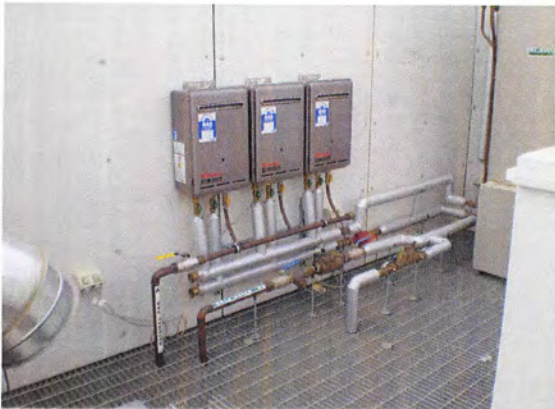
Gas Fired Instantaneous Hot Water System
