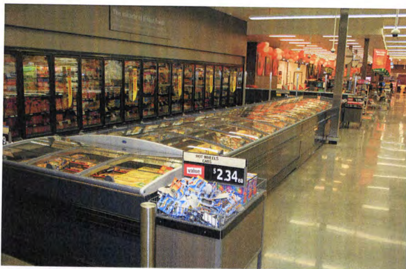
Lights off on Glass Door Freezers – Woolworths Norbrik Also, Wide Island Freezer Lids
