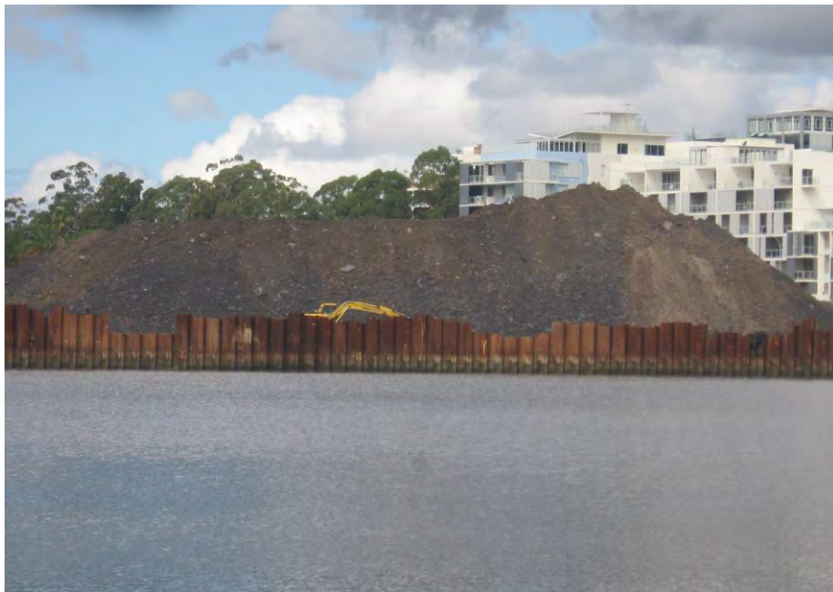
Plate 6: Remediation site on eastern (Rhodes) side of subject site.
