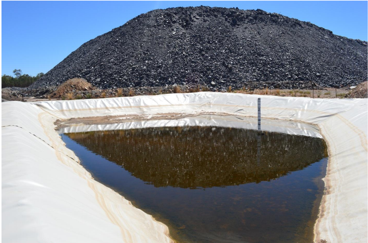
Plate 1 Southern Waste Rock Emplacement Leachate Management Pond
