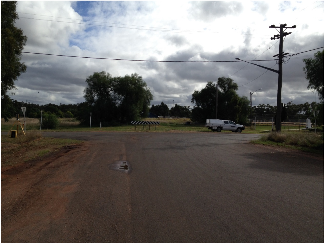
Plate 11: Nymagee-Hermidale Road and Nyngan Street intersection looking north from Nymagee Street
