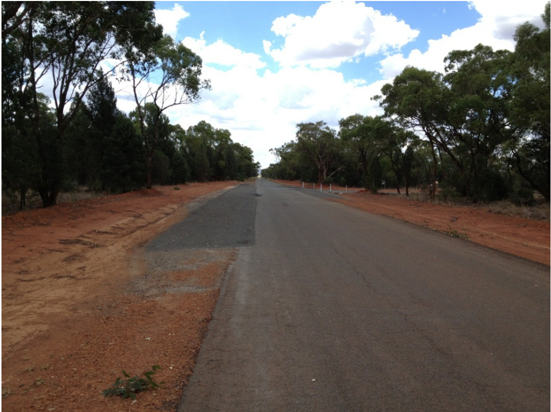
Plate 1: YTC Site Access looking north along Burthong Road
