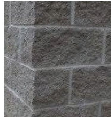
CBP - Concrete Block Work-Paint Finish
