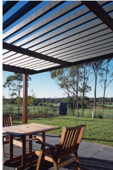
TBP- Timber Pergola
