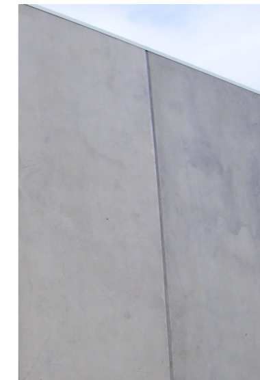
COP - Precast Concrete
