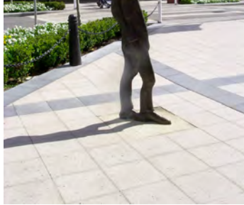
Concrete unit pavement
