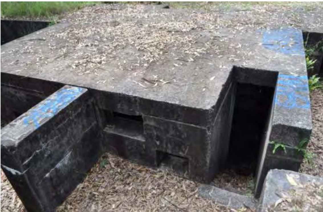
Figure 5.7: Wangi Wangi anti-aircraft battery command centre. Source: EJE Architecture, February 2011
