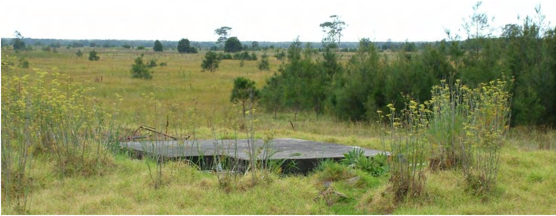
Figure 3.21: The Command Post Source: EJE Architecture 2011
