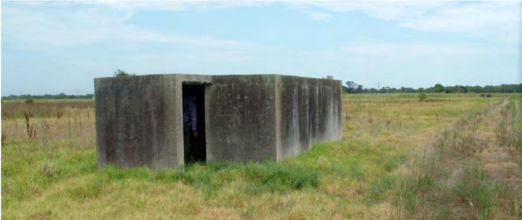
Figure 3.24: Ammunition Magazine Source: EJE Architecture 2011
