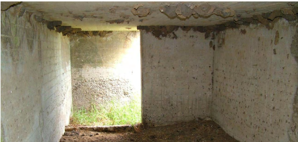
Figure 3.26: Ammunition Magazine Source: EJE Architecture 2011
