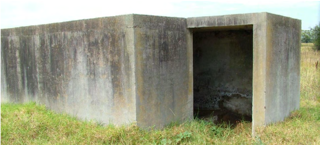
Figure 3.25: Ammunition Magazine Source: EJE Architecture 2011
