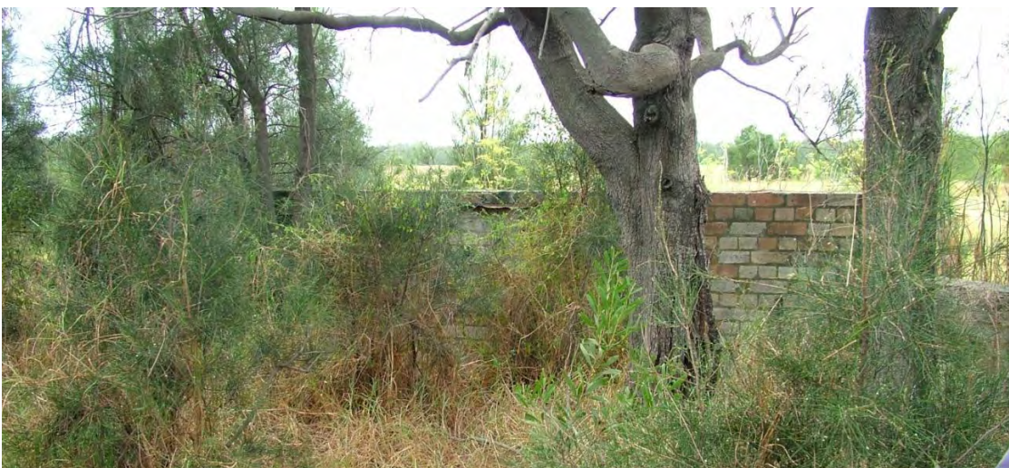
Figure 3.20: Gun Emplacement (G4) Source: EJE Architecture 2011
