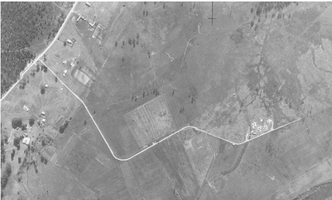
Plate 29 Aerial photograph showing the site in 1944 shortly after construction of gun emplacements and ammunition shelters
