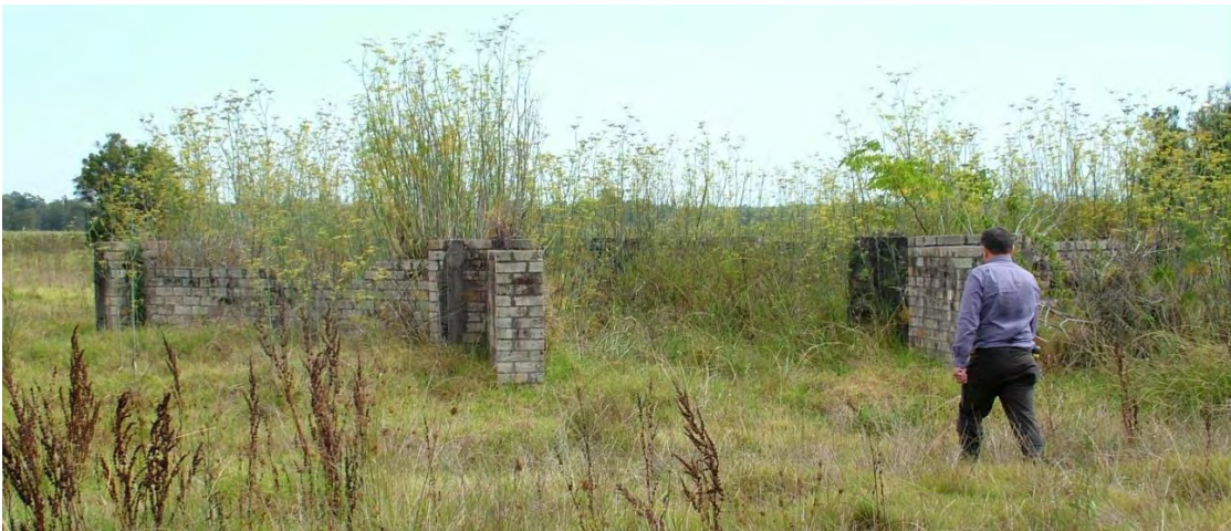
Figure 3.19: Gun Emplacement (G3) Source: EJE Architecture 2011
