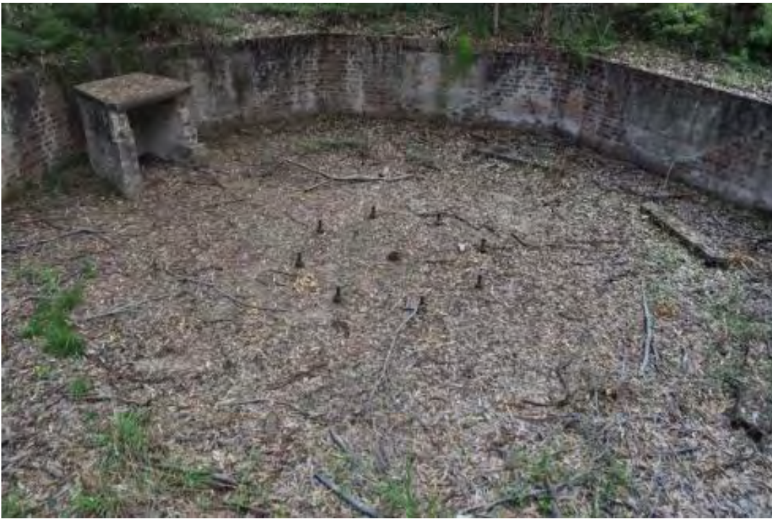
Figure 5.6: Wangi Wangi anti-aircraft battery gun emplacement. Source: EJE Architecture, February 2011
