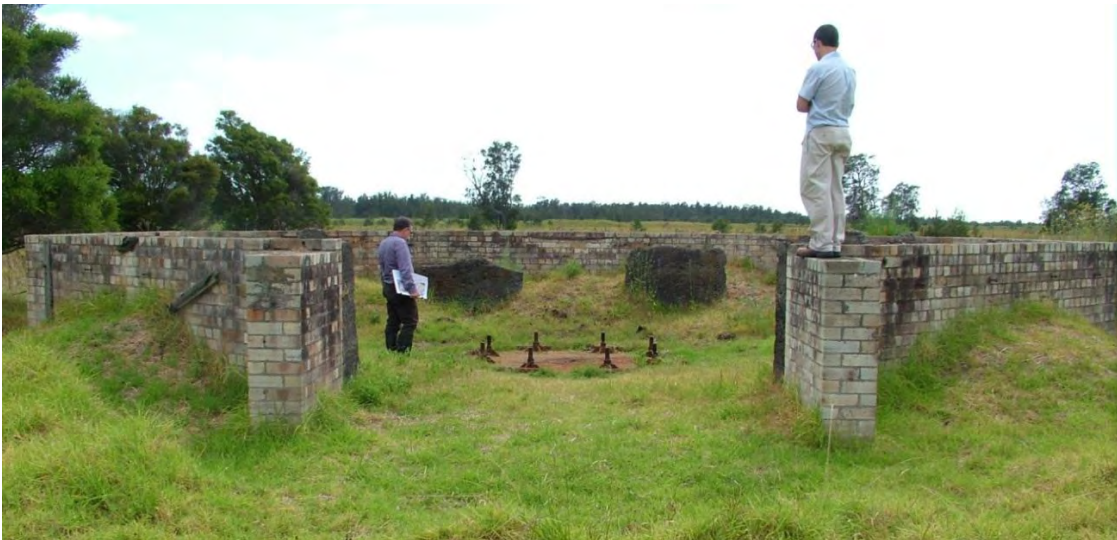
Figure 3.16: Gun Emplacement (G1) Source: EJE Architecture 2011
