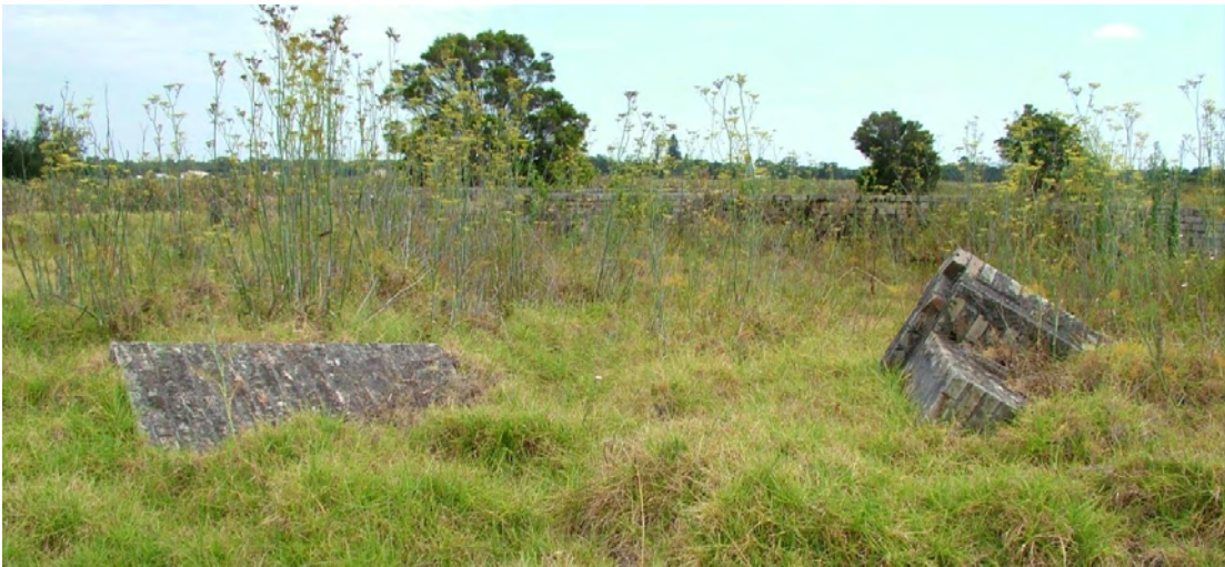
Figure 3.18: Gun Emplacement (G2) Source: EJE Architecture 2011
