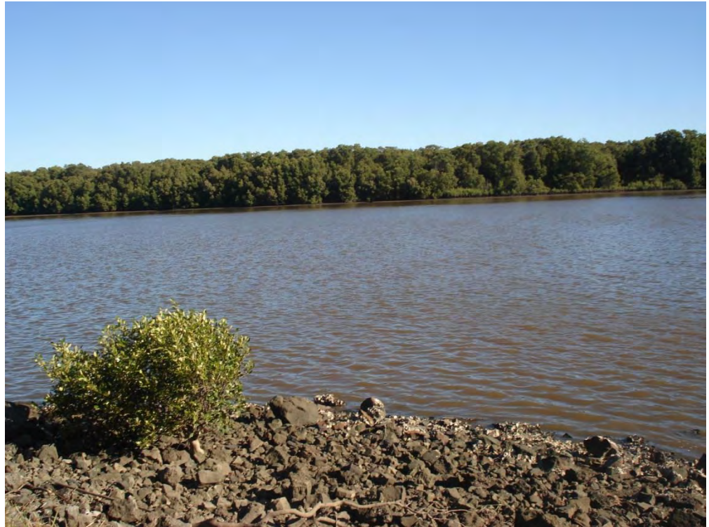
Plate 7. Rock revetment works along the Study Site foreshore on the Hunter River
