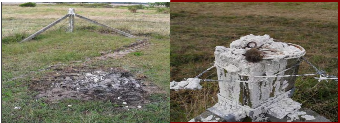
Photo 46 & 47 – Burnt refuse at ground surface comprising glass, metal, ash, gravel and white substance (looking south-east). White substance on fence with dead mouse.
