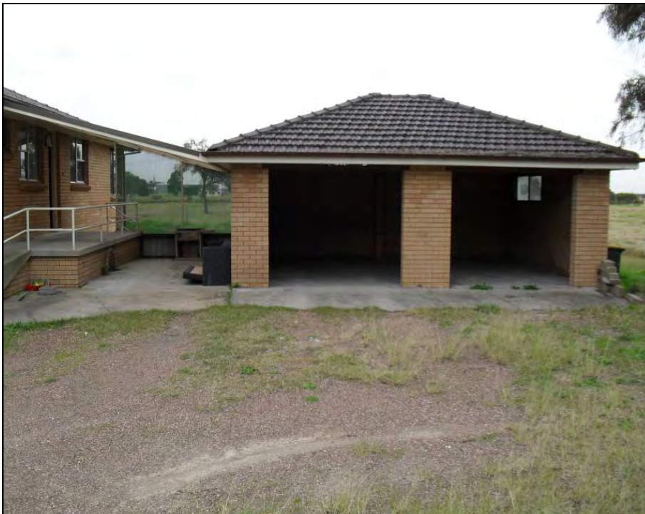
Photo 25 – Brick garage adjacent vacant brick residence with gravel driveway in foreground (looking east)
