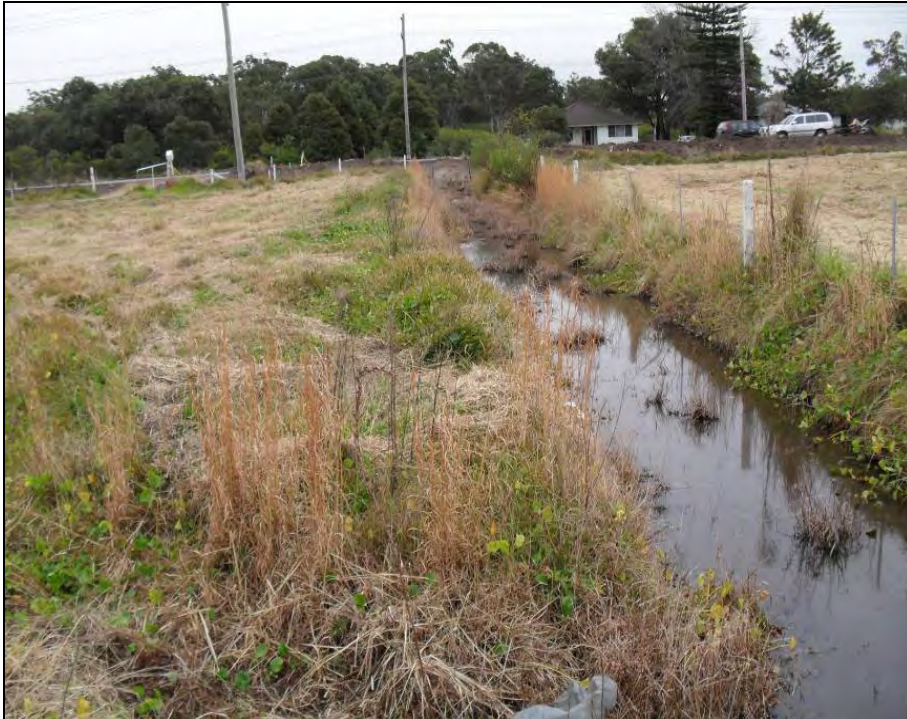
Photo 4 – Drain about 2 m wide in northern portion of site (looking north). Some orange algae and waxy film on surface, plus bricks, concrete observed in drain.
