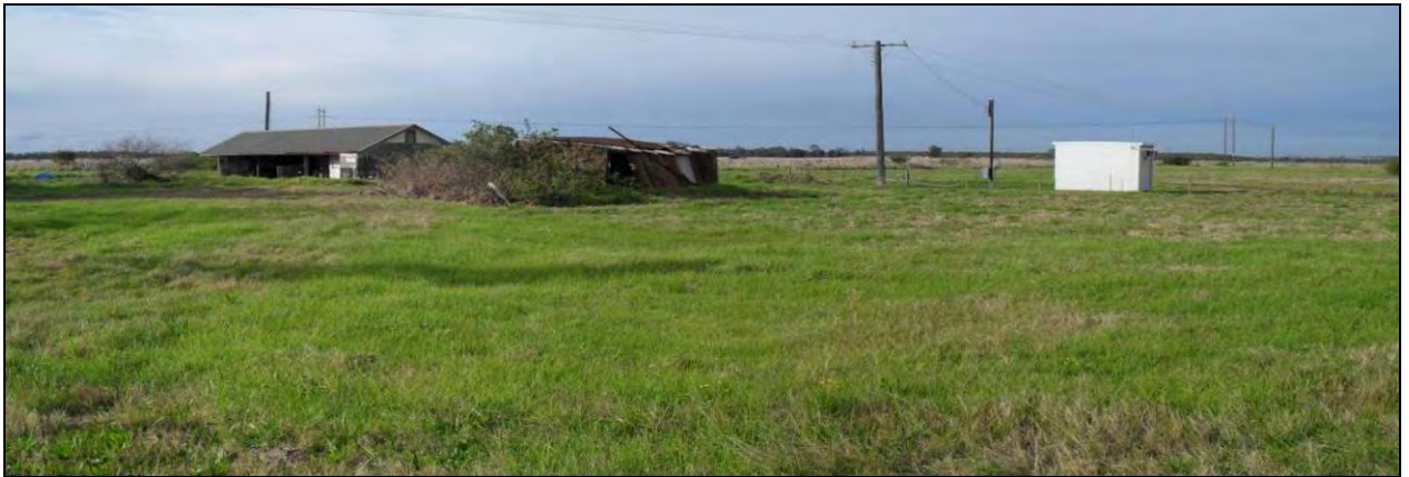
Photo 24 – Vacant sheds constructed from fibro sheeting, bricks, corrugated iron, timber. Fibro sheeting fragments, gas bottles, 44 gallon drums, scrap metal etc observed around sheds (looking south east)
