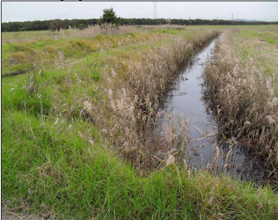
Photo 7 – Drain with adjacent stockpiled spoil (looking west towards Hunter River)
