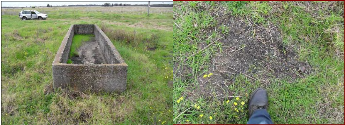
Photos 39 & 40 – Rectangular concrete trough. Ash fill observed adjacent to trough.
