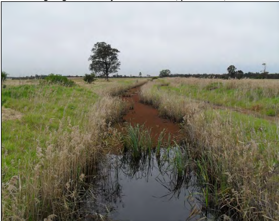
Photo 5 – Drain about 4 m wide and 2 m deep in south-western portion of site. Red algae observed at surface. Spoil stockpiled to the south of drain.
