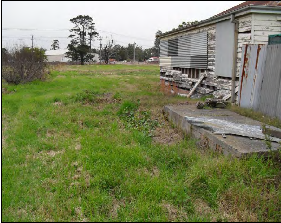
Photo 43 – Septic tank and concrete/brick chamber adjacent dwelling (looking north)
