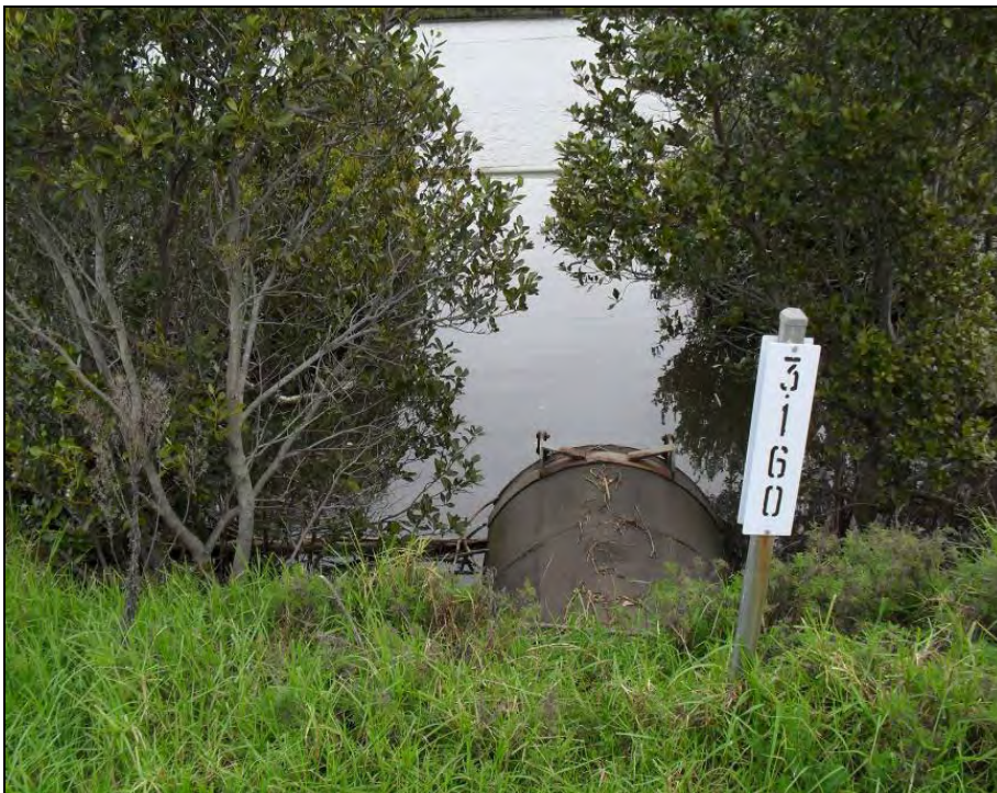
Photo 51 - Drain discharge point into Hunter River (looking south-west)
