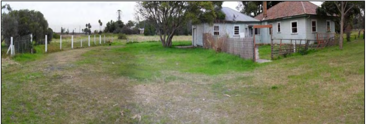
Photo 22 – Vacant dwelling and rear garage (looking west). Fibro observed around bottom edge of brickwork. Some ash filling observed in gravel driveway (left).
