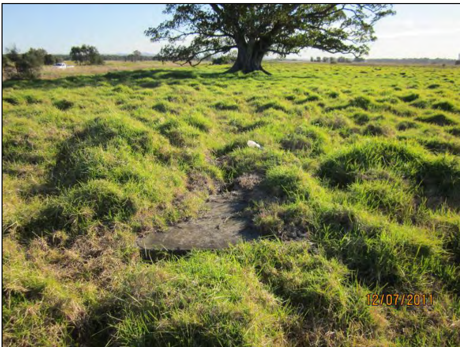
Photo 9: Septic tank with broken concrete lid in the southern portion of the site, thick grassed covered field in background, drain with thick reed cover (left)
